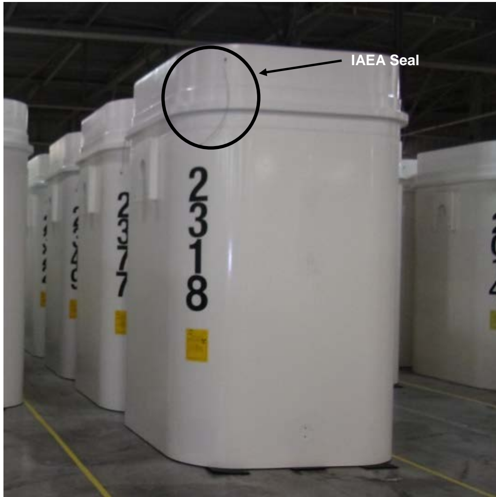
Figure 19: DSCs in Storage with IAEA Wire Seals
